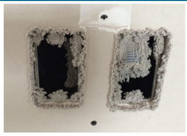
Figure 4. Photo showing untaped network access points on an interior wall with significant deposition
