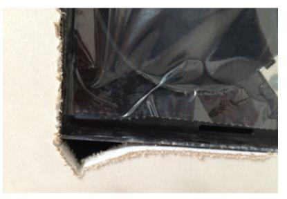
Figure 5. Photo showing hole near ventilation supply duct that was not expected to be sealed by the aerosol process and left uncovered to reduce the time required for setup
