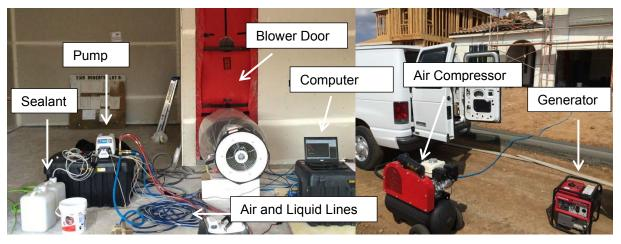
Figure 7. Primary equipment used for aerosol sealing installation
