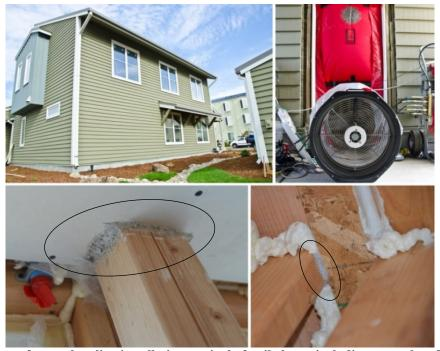
Figure 2: Photos of aerosol sealing installation on single-family home including examples of seals formed.
