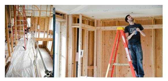
Figure 3: Photos of Honda Smart Home before aerosol envelope sealing application.
